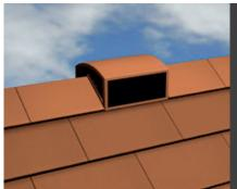
Modern houses generally later than 1960 often have a pre-cast concrete chimney system, identifiable by a rectangular box section flue and a terminal, as illustrated in the picture above.
