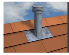
Either an older house where the existing chimney has been lined by a proprietary steel flue or a newer house with a steel flue built in. This chimney type is identifiable by a 5" (130 mm) diameter flue and a steel flue terminal.
